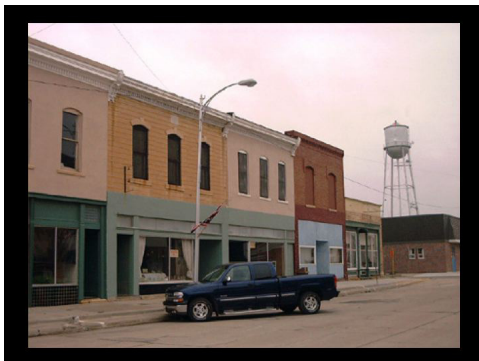
Slide #7 - No name on water tower
